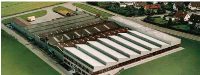
Häfele Production Plant Jettingen, Germany
